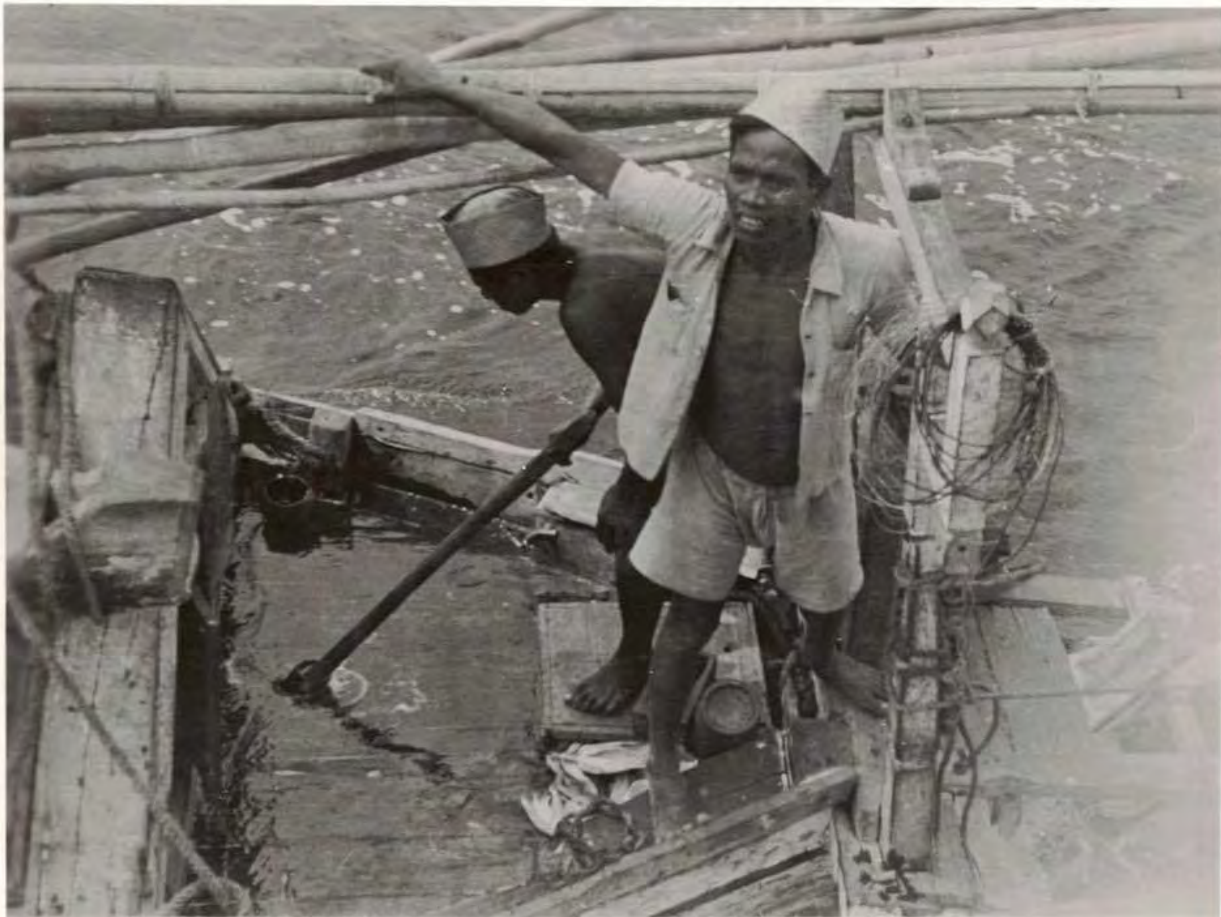
10 BILGE PUMP A LA SAMBAN
