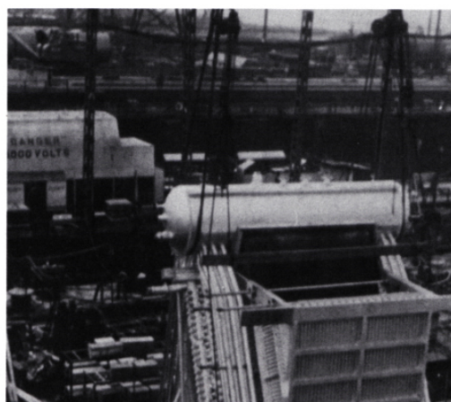
One of eight USS RANGER boilers being lowered into position
