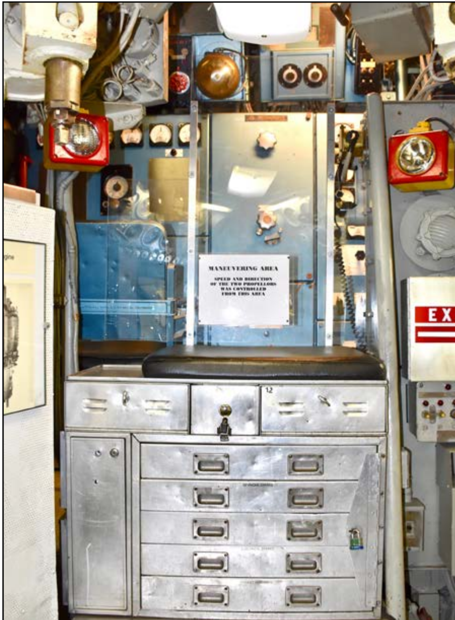
Entering the engineering/propulsion spaces, facing aft. One sees the large equipment cabinet and the elevated maneuvering area immediately behind it. Notice that the equipment cabinet has a padded bench top.
