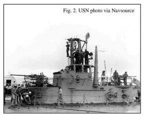
provide excellent platforms for mounting of additional anti-aircraft guns, but it provided locations for additional radar masts and auxiliary antennas. Three heavy I-beams rose up vertically on either side of the conning tower, then turned 90° inwards to provide structural support for the periscopes and platforms for lookouts. Once the plating was removed from around these beams, the visual effect gave rise to the *Gatos* being nick-named the "Covered Wagon Boats" (Figure 2).
