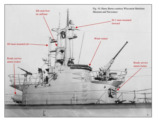
Figure 10 is an excellent August 1944 photo of *Loggerhead* in her Type 2 configuration. Very evident are the typical EB design bow-tie shears stiffeners, two additional ready service ammo gun tubs under the fore and aft fairwater gun decks, and the LF loop antenna between the shears. She has the heavy Mk 3 40 mm forward and a 20 mm Mk 10 gun aft, a typical outfit for Manitowoc boats of this period. Except for the gun armament and the SJ position, notice the overall similarity
