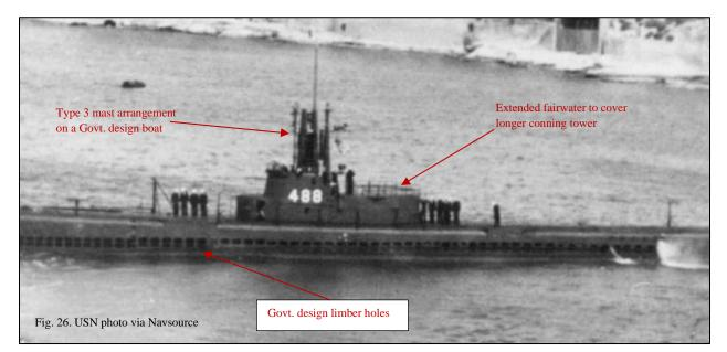
arrangement. *Sarda*, commissioned in 1946, is the only Government design boat with an EB style Type 3 mast configuration. The longer conning tower, while seemingly a good idea, was not repeated due to new post-war thinking that led to the integration of the attack center into the control room. This idea first showed up in practice in the new fast attack boats of the *Tang* and *Darter* classes in the early 1950's, which did away with a conning tower for the first time.
