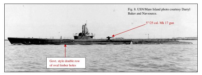
*Spadefish* (SS-411) is shown in Figure 8 off Mare Island on 11 May 1944. Even though she is in her as-built Type 1 mast configuration, she is sporting the 5"/25 caliber Mk 17 gun in the aft position. She was the first boat to be built with the heavier gun.
