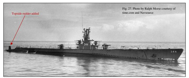
below water rudder. Not as successful as first hoped, it was not a widespread modification. The Type 3 *Cobbler* is shown in Figure 27 in 1948 with this rare modification; the additional topside rudder is just visible on the far left.
