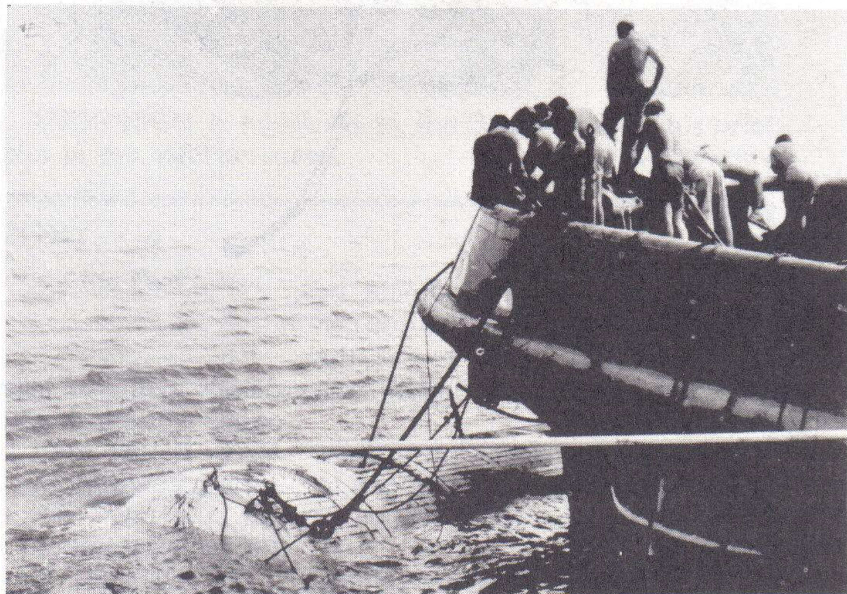
CREWMEN ON THE PRESERVER lower the after-lift pontoon in preparation for the final lift.
