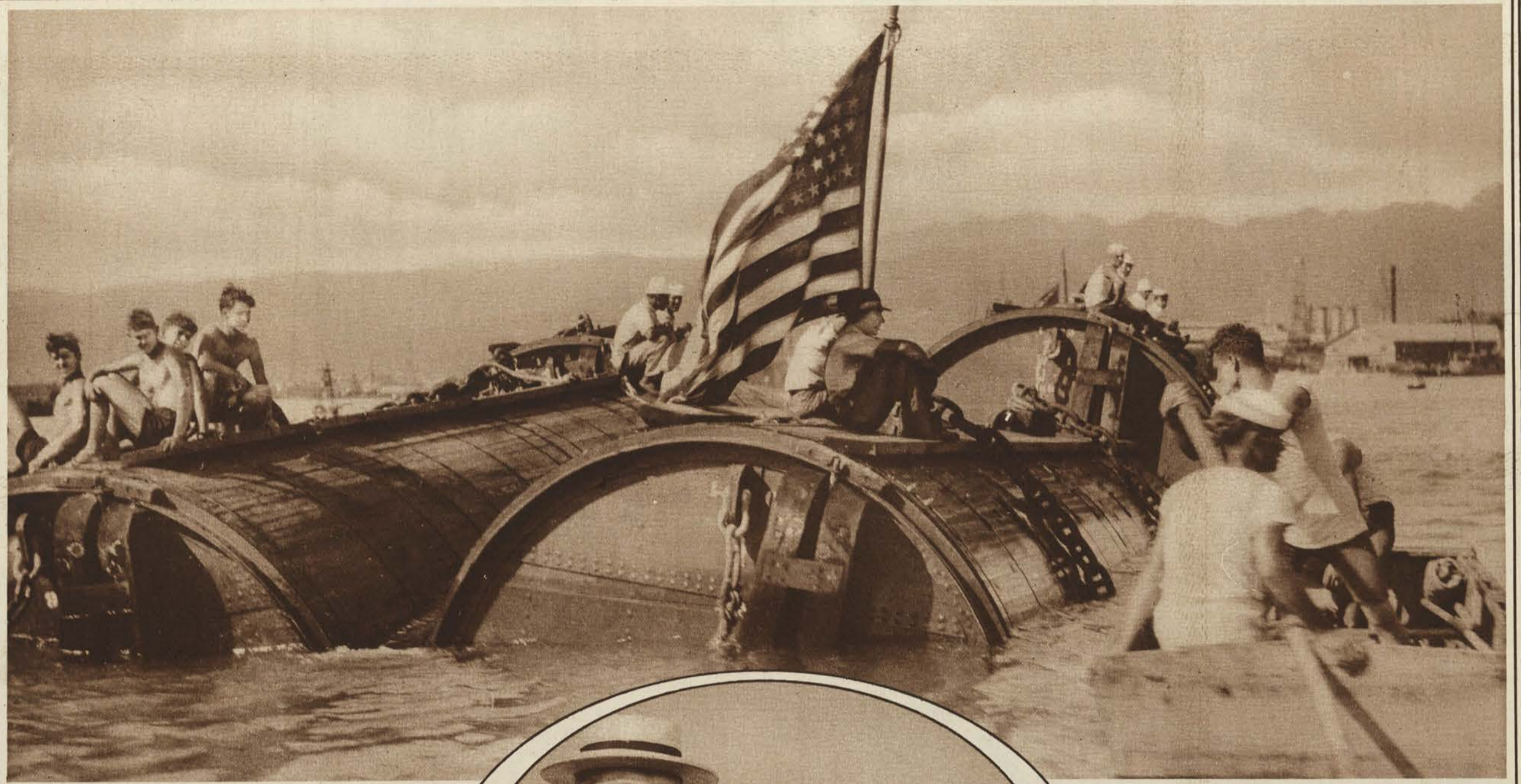
The United States Submarine F-4, Which Sank Off Honolulu with the Loss of All on Board, Towed Into Honolulu Harbor, Supported Six Feet Below the Surface by Huge Pontoons. The Sailors Have Hoisted the Stars and Stripes Lashed to an Oar. (Photo from J. M. Cummings.)
