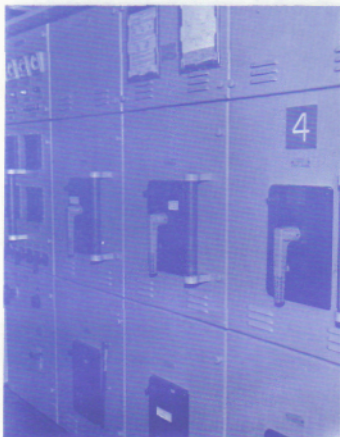
#1 EMERGENCY DIESEL SWITCHBOARD 2-29-2Q
