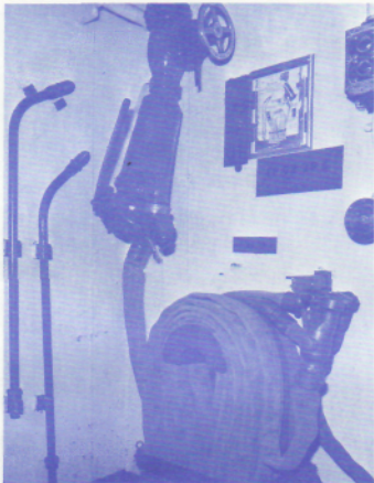
FIRE STATION AND HOSES WITH APPLICATORS 02-00H-OQ
