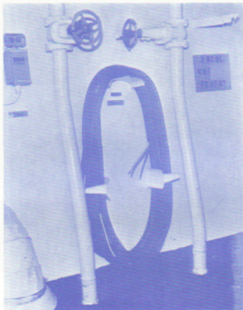
CABLE RACK CASUALTY POWER SUPPLY SYSTEM 2-89-2
