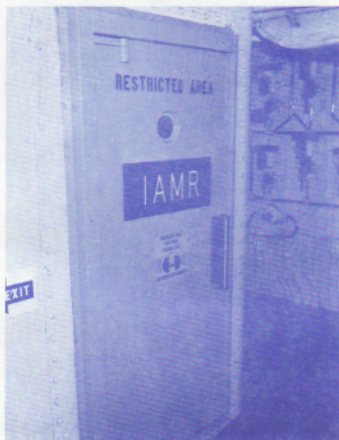
#1 AUXILIARY MACHINERY ROOM 1 AMR (EXTERIOR) 2-102-3
