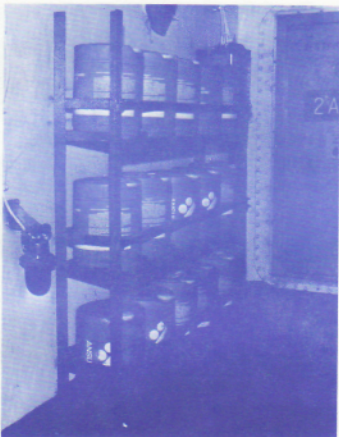
AQUEOS FILM FORMING FOAM (AFFF) 600 GALLON STATION 2-139-3
