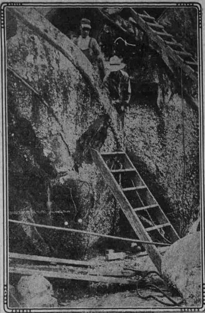
N the work of cutting up the remains of the battleship Maine in Havana harbor the oxyacetelene gas-torch is being used very effectively. With this device the tangled wreckage is quickly cleared away and openings are easily cut through steel plate.
