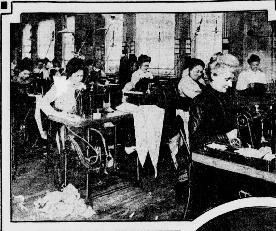
A BUSY CORNER OF THE MACHINE ROOM.
