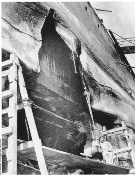
The battleship Nevada , undergoing repairs at Pearl Harbor Navy Yard in early 1942, displays the torpedo damage she sustained.
