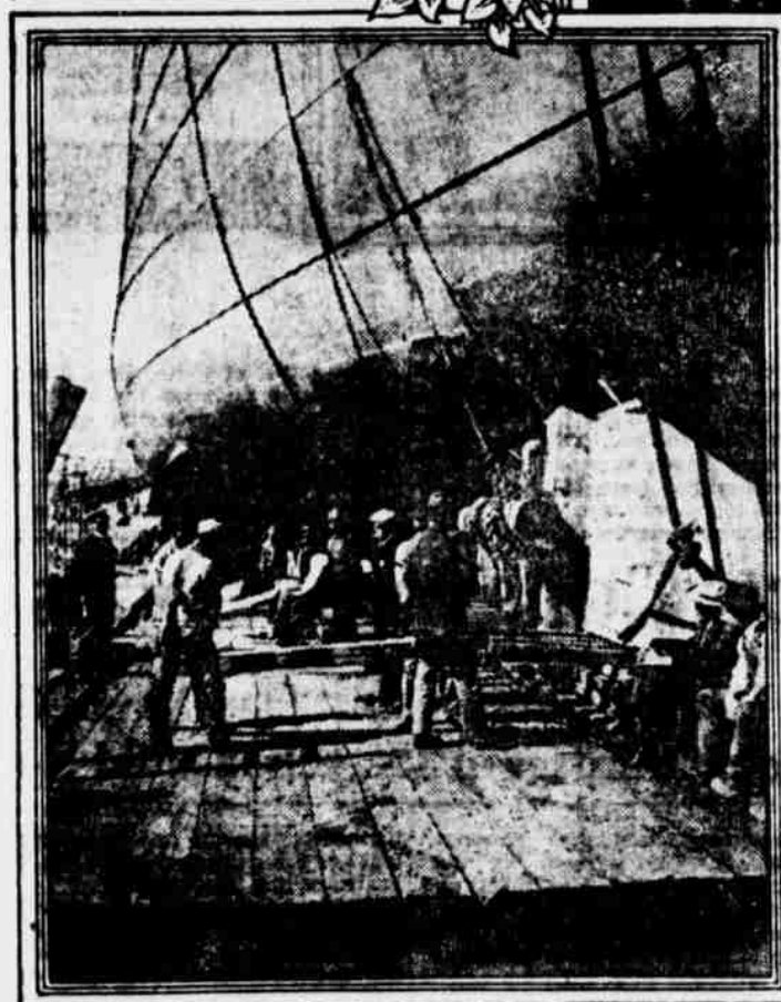
FINISHING THE "WEDGING UP" ONLY THE SAWING OF THE SOLE-PIECE, AND BREAKING THE BAPTISMAL BOTTLE ON THE SHIP'S STEEL STEM INTERVENE BEFORE THE GREAT CRAFT SLIDES WATERWARD
