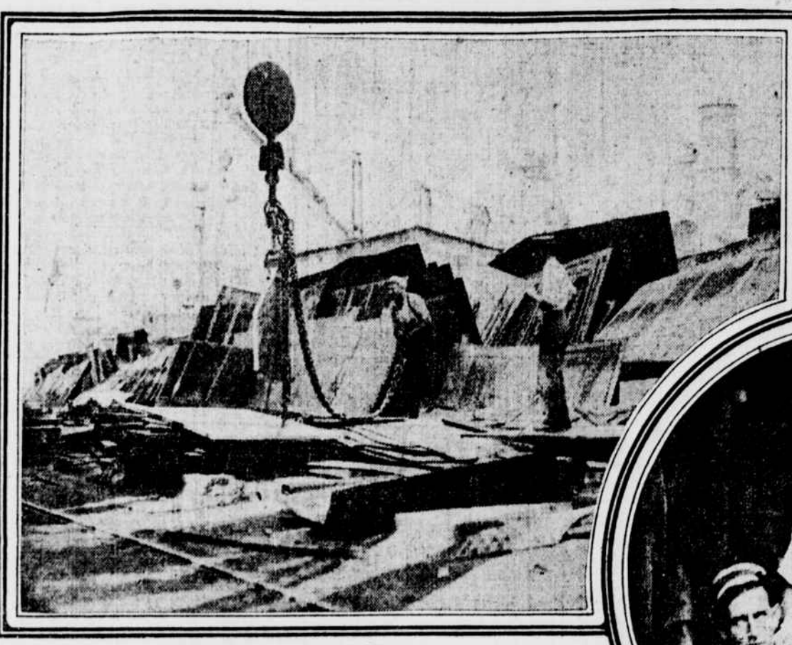
Hoisting the Steel Plates
