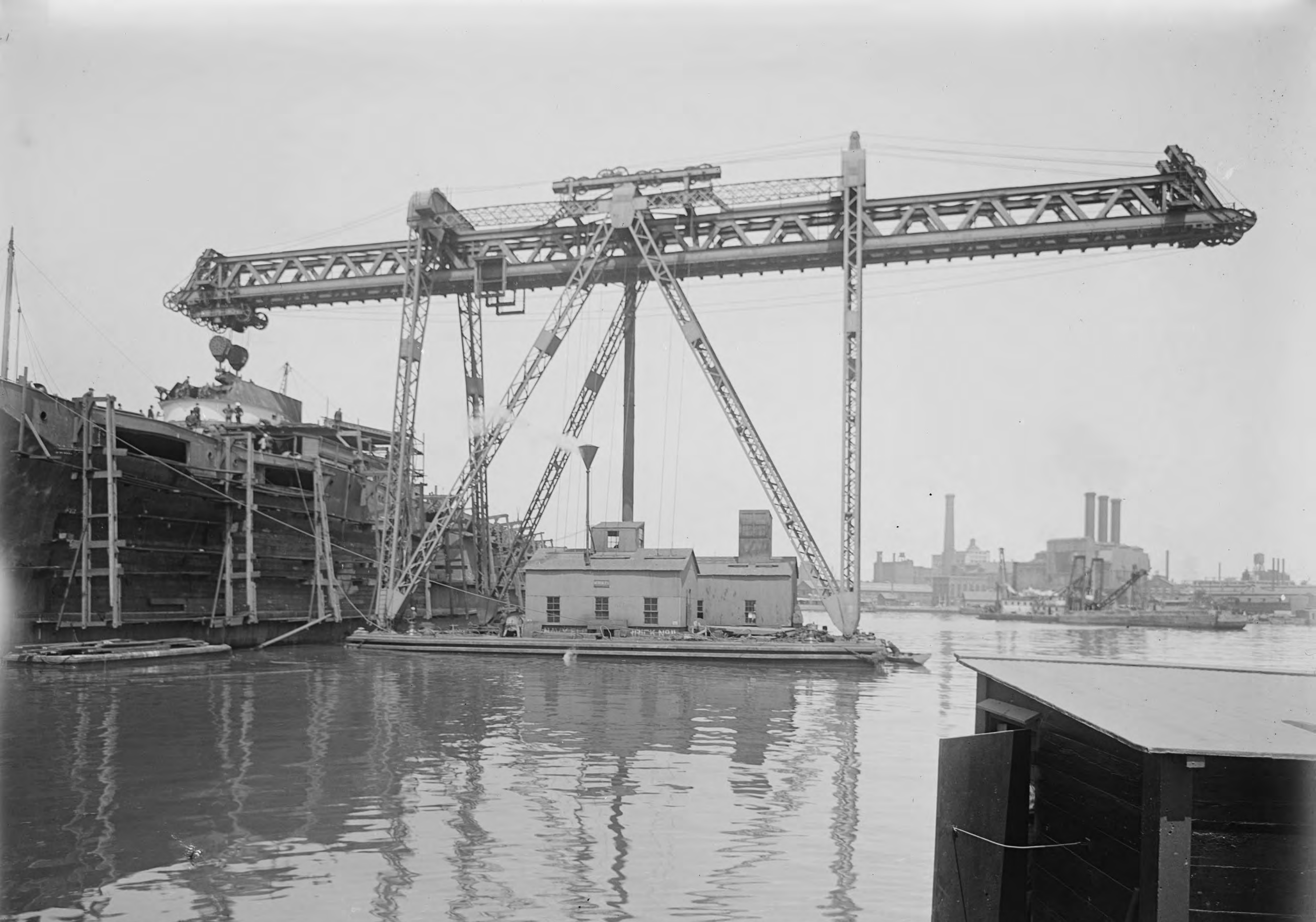
F604N85. NAVY YARD, NEW YORK, 5-8-13, CRANE HERCULES PLACING TURRET NO. 2 (WT. 220,000 LBS) IN POSITION ABOARD U.S.S. NEW YORK. LOWERING TURRET.
