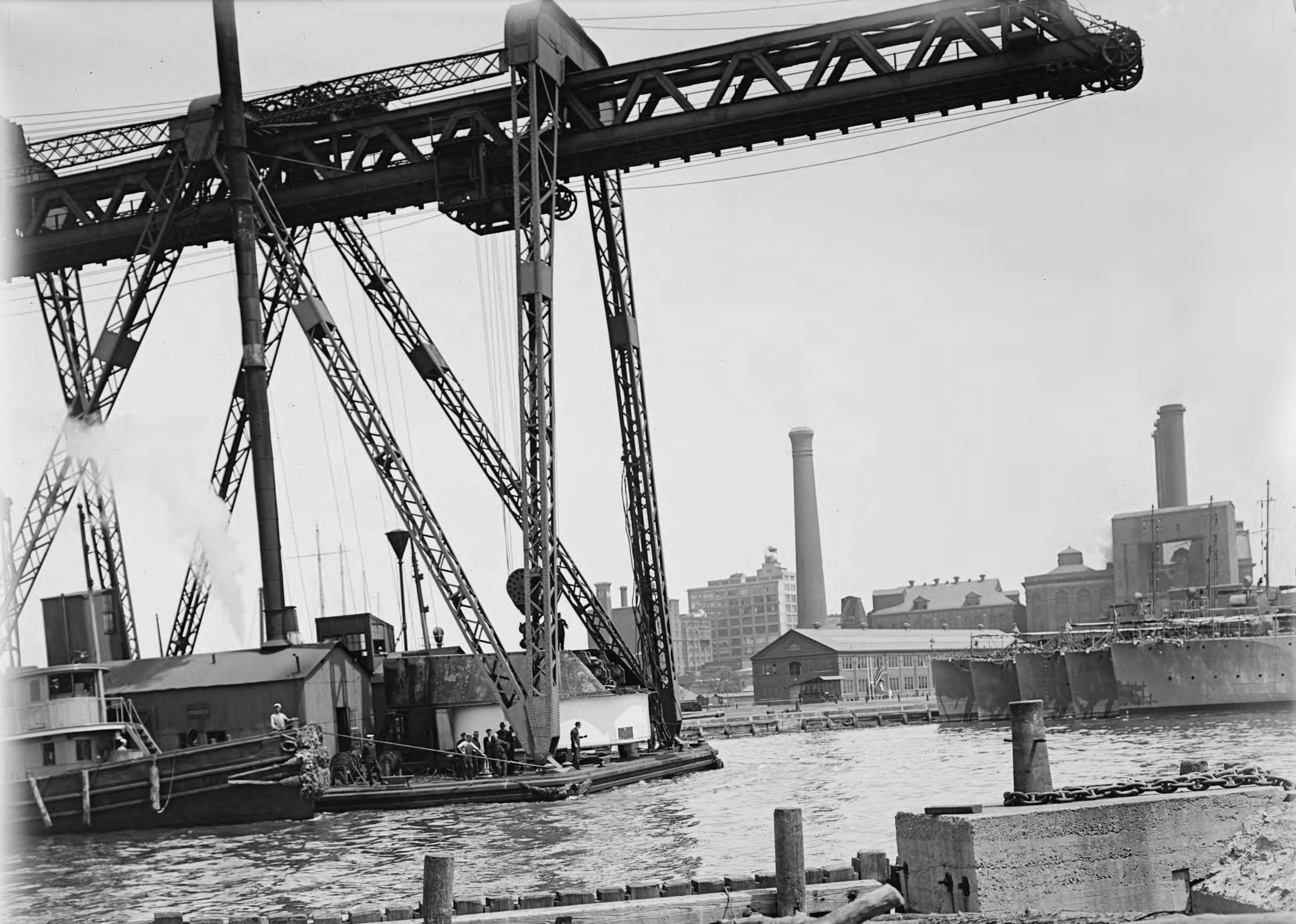
F604N84. NAVY YARD, NEW YORK, 5-8-13, CRANE HERCULES WITH TURRET NO. 2 (WT. 220,000 LBS.) U.S.S. NEW YORK IN TOW OFF ORDNANCE DOCK.
