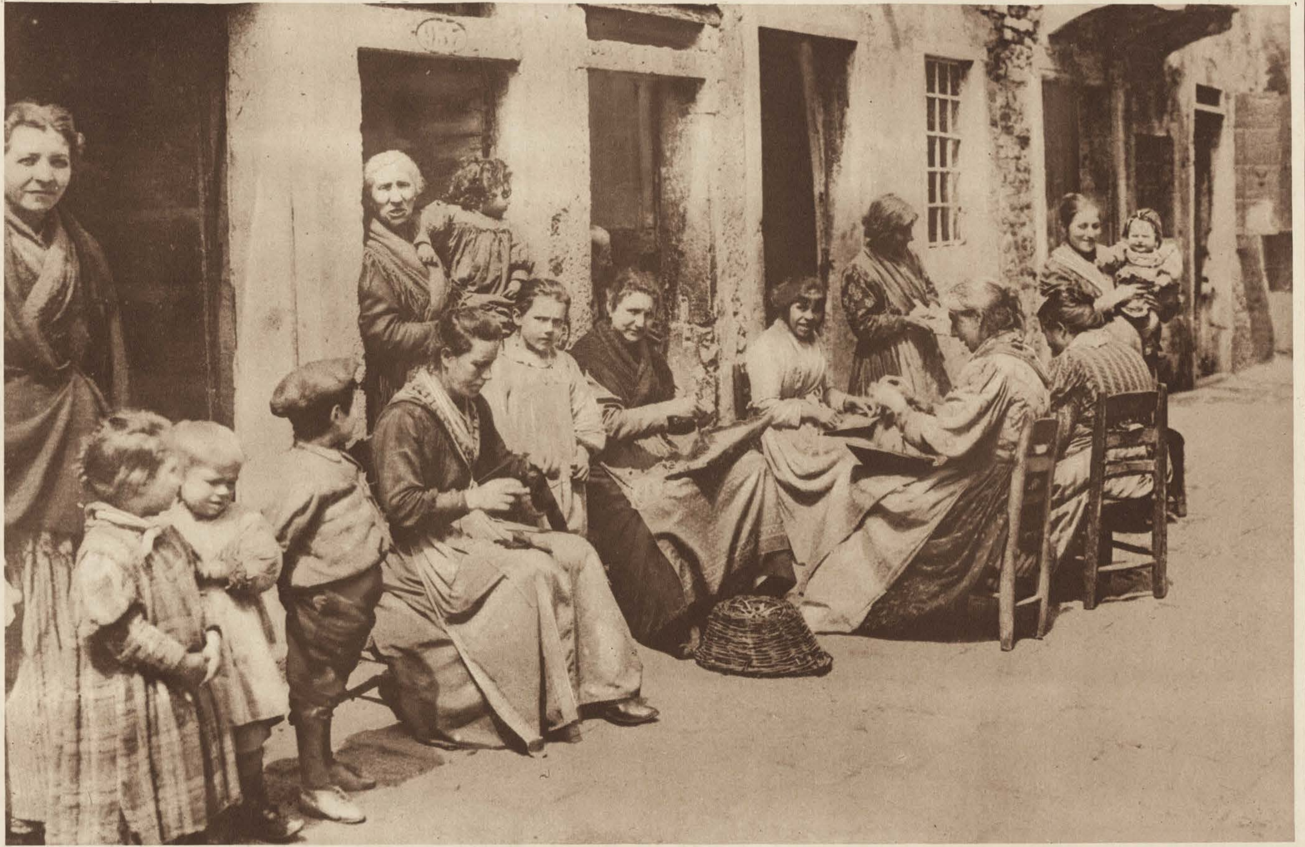
WOMEN AND CHILDREN BEFORE THEIR DOORS IN THE ONCE HAPPY TOWN OF AVEZ ZANO, ITALY, THE CENTRE OF THE EARTHQUAKE OF JAN. 13, WHICH COST 30,000 LIVES AND $60,000,000 IN PROPERTY (Photo by American Press Assn.)
