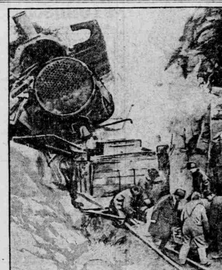
A DEATH-FILLED GAP—Two trains met head-on in this gap on the Philadelphia and Reading line at Woodmont, Pa. One locomotive leaped the loop. Cars were telescoped. Gas tanks exploded. More than 20 commuting residents of nearby towns were killed and 30 injured.
