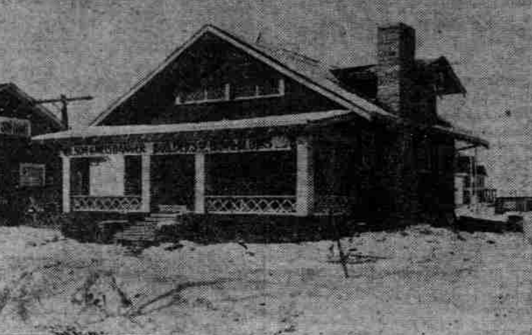
Bungalow No. 4, Just Completed at the Corner Hutton and College Avenue.
