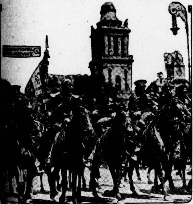
This picture of a detachment of federal cavalry was taken during a parade of the troops through the streets of Mexico City, at the height of the Huertista movement over the breaking out of hostilities with the United States.
