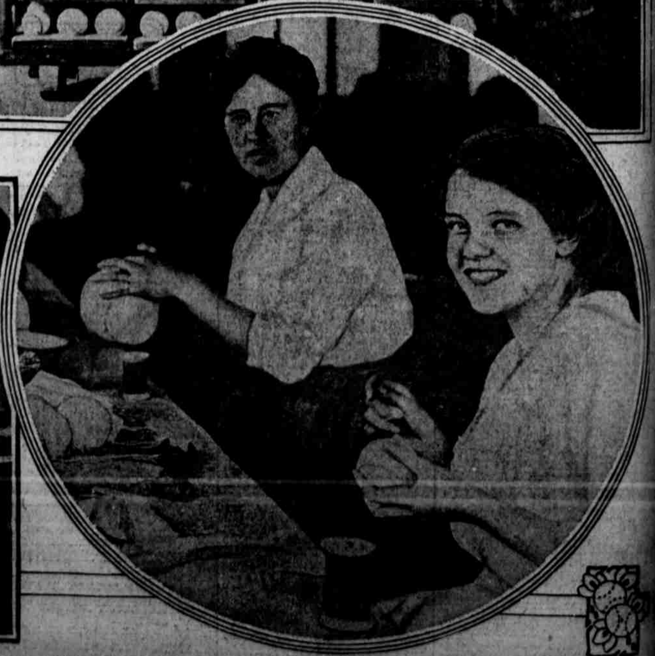
FIRST PHOTOGRAPHS EVER PUBLISHED IN A NEWSPAPER OF BIG-LEAGUE BASEBALLS IN THE PROCESS OF MANUFACTURE Sewing the horsehide covers on by hand.
