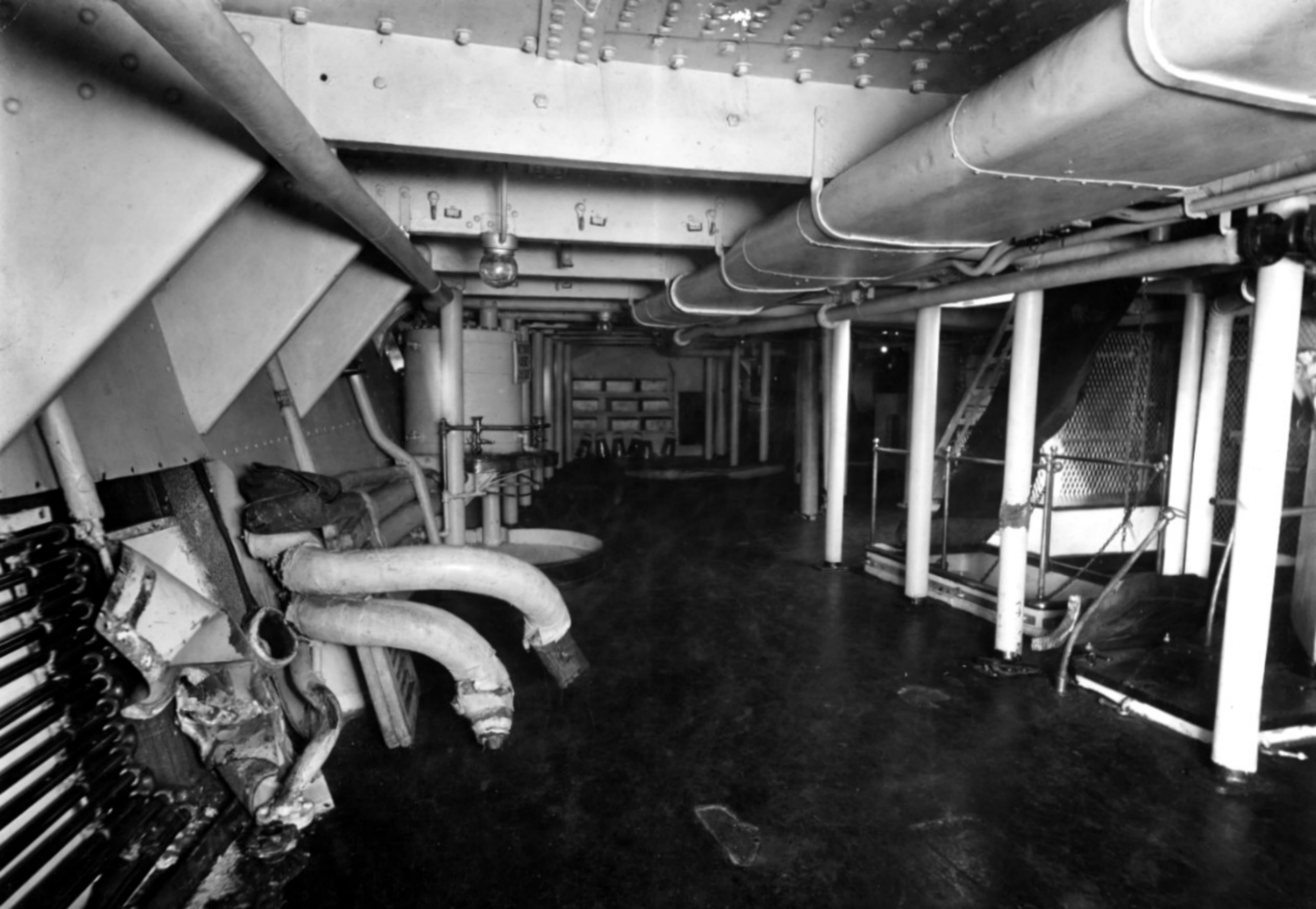
U.S.S MICHIGAN. NAVY' YARD PHILA. PA SEP 25-1916. PORT SIDE BETWEEN UPPER & MAIN DECK AT ABOUT FROM 22 & 23. MAIN DECK VIEWED FROM. IN BOARD & SLIGHTLY ALOFT INJURY.
