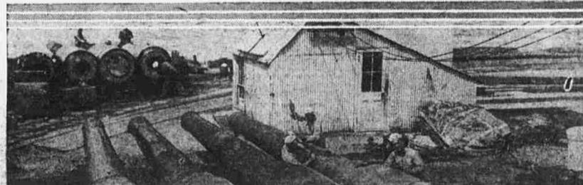
Defects having been found in her main battery, these new 12-inch guns are being placed aboard the Michigan, which is undergoing repairs at League Island under rush orders.
