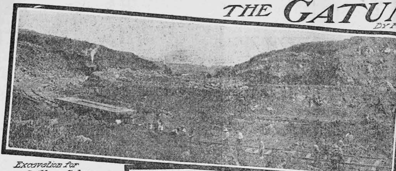
Excavation for Spillway Gatun
