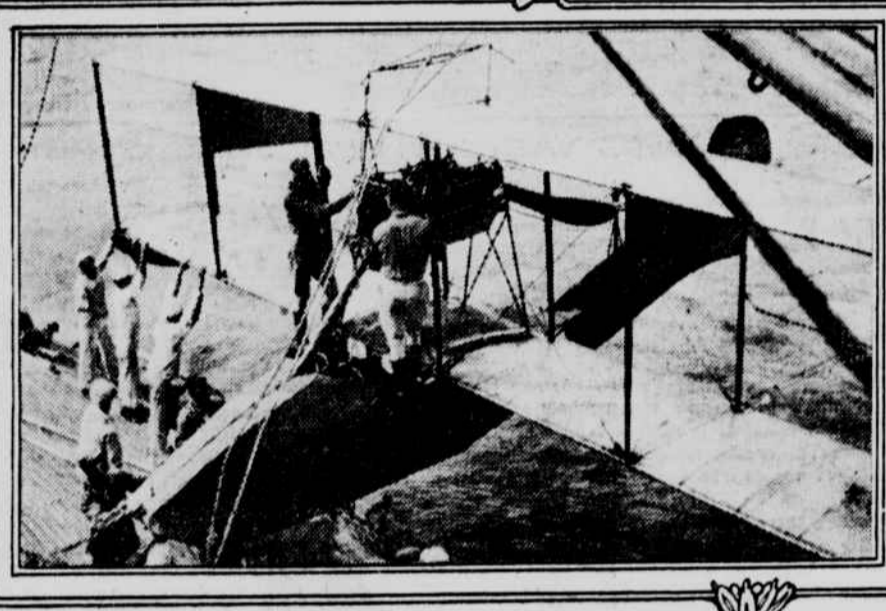
SAME LIFTED FROM DECK TOWERS AT LEFT
