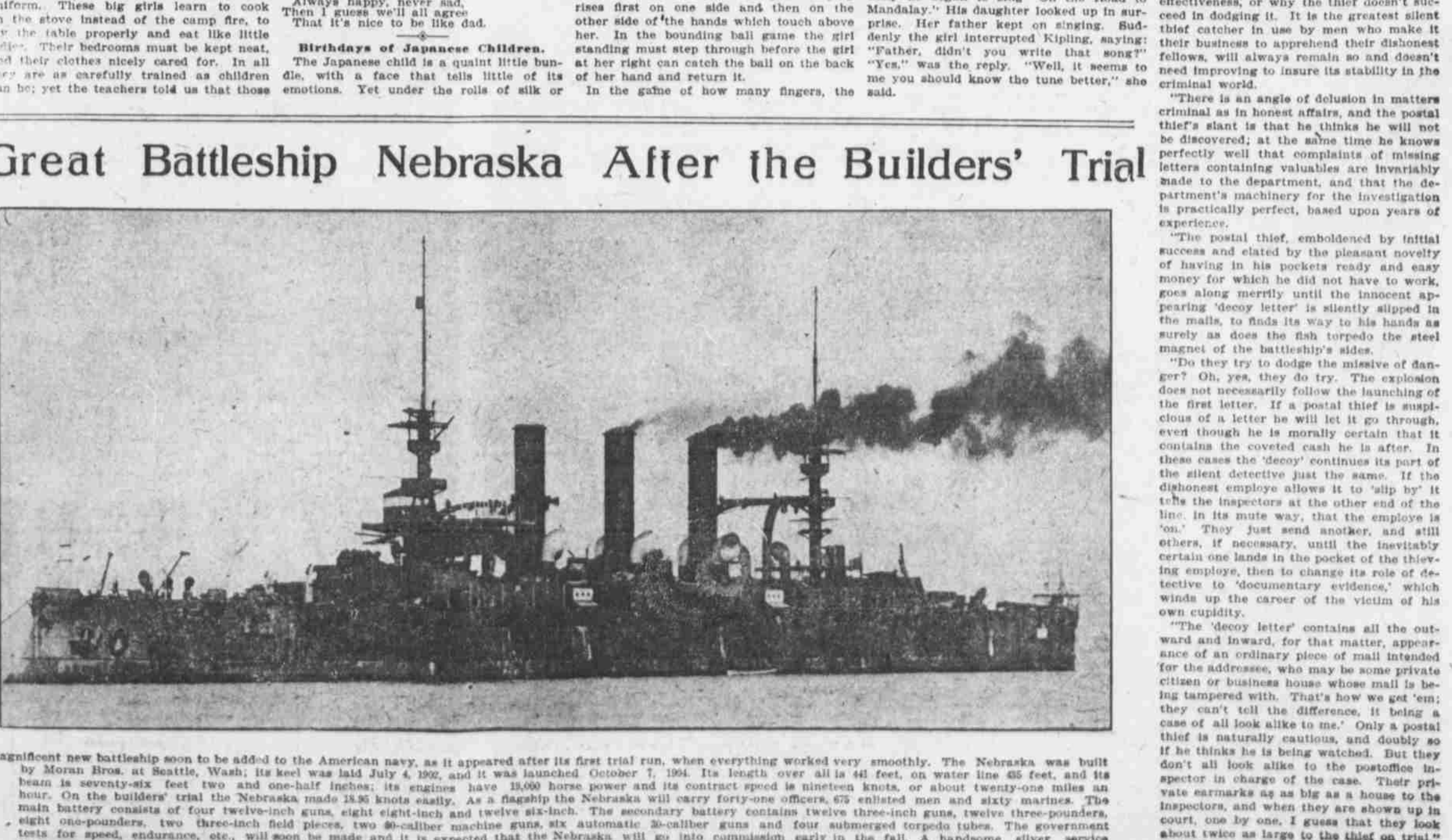
Magnificent new battleship soon to be added to the American navy, as it appeared after its first trial run, when everything worked very smoothly. The Nebraska was built by Moran Bros., at Seattle, Wash.; its keel was laid July 4, 1902, and it was launched October 1, 1904. Its length over all is 441 feet, on water line 35 feet, and its beam is seventy-six feet two and one-half inches; its engines have 15,000 horse power and its contract speed is nineteen knots or about twenty-one miles an hour. On the builders' trial the Nebraska made 18.85 knots easily. As a flagship the Nebraska will carry forty-one officers, 675 enlisted men and sixty marines. The secondary battery consists of four twelve-inch guns, eight eight-inch and twelve six-inch. The automatic 3-inch machine guns, six automatic 2-inch machine guns, and four submerged torpedo tubes. The government tests for speed, endurance, etc., will soon be made and it is expected that the Nebraska will go into commission early in the fall. A handsome silver service has been purchased by the state of Nebraska for presentation to the ship.—Photo by Webster & Stevens, Seattle.
