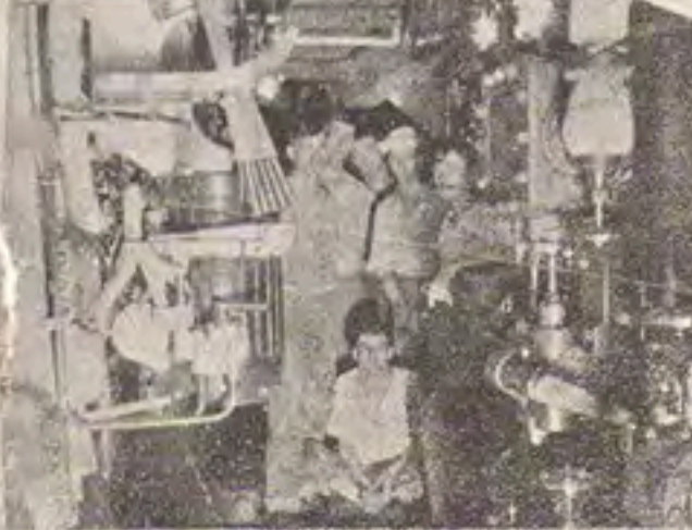
THE PORT ENGINE ROOM.
