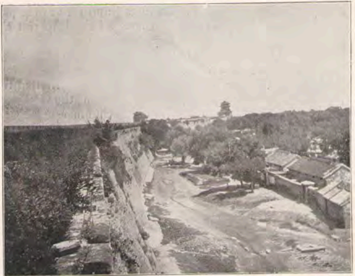
THE NORTH WALL OF PEKING, LOOKING TOWARD THE EAST.
