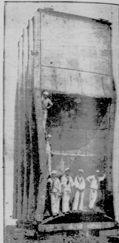
EFFECT UPON THE TARGET OF THE TORPEDO WHICH SANK IT.
