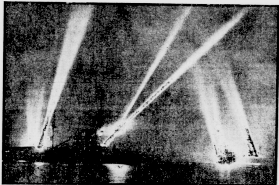
SEARCHLIGHT PRACTICE ON A FLEET OF WARSHIPS. One of the features of the manoeuvres near Provincetown, Mass., was the practice with searchlights for training the sailors to detect the approach of torpedo boats and submarines and to discover the best location for the searchlights on the new fire control masts.
