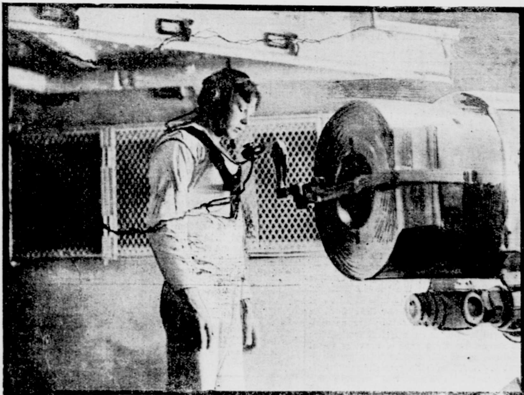
GUNFIRE IS DIRECTED FROM THE FIRE CONTROL MAST BY TELEPHONE. The noise of the guns and machinery drowns verbal orders.
